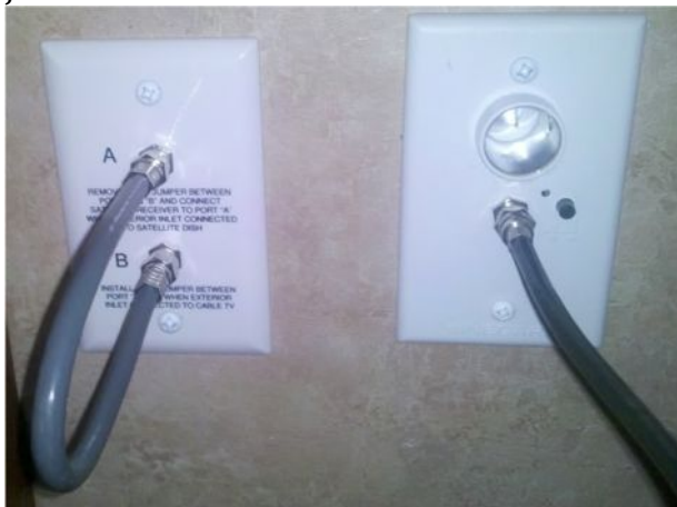
[illustration 2] (left) Satellite / Cable connections and jumper (right) power antenna / television connection.
